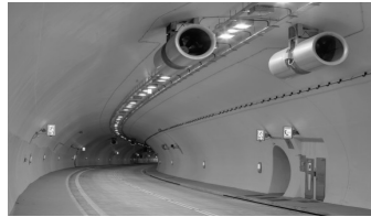
Figure 6. Longitudinal ventilation
